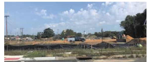
Wawa is under construction on Rt. 49
